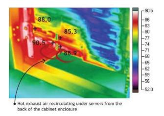
Open spaces at the bottom of the cabinet and between the mounting rails and side of the cabinet allow hot exhaust air to re-circulate to the front of the cabinet where it is ingested by IT equipment. Sealing these openings will help to ensure conditioned air is delivered properly to IT intakes.
